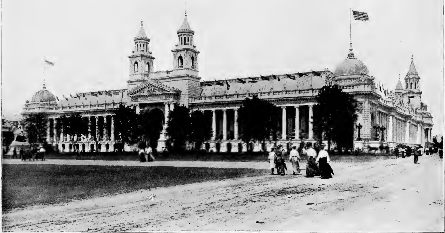
PLAZA FRONT OF PALACE OF VARIED INDUSTRIES.
